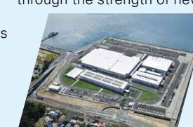
Hiroshima Plant of U-Shin Ltd.
